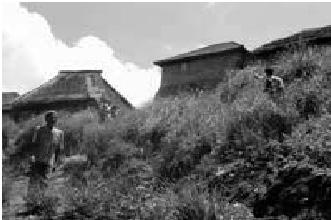
Photo 2 Vetiver stabilizes sandy slope
